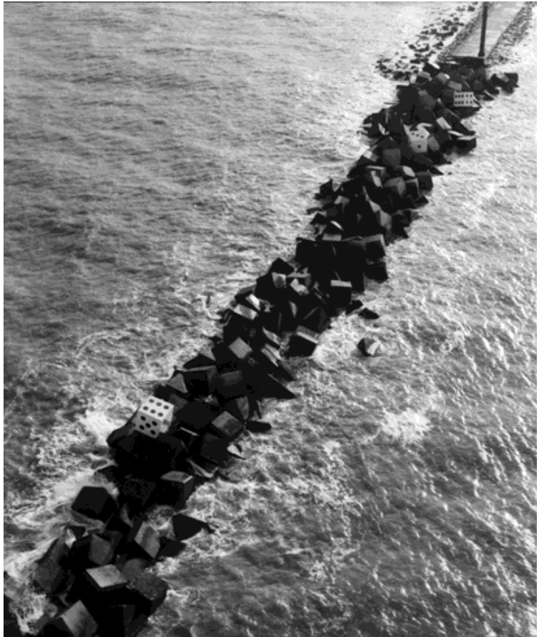
Dice blocks on breakwater Hook of Holland (courtesy Rijkswaterstaat)
