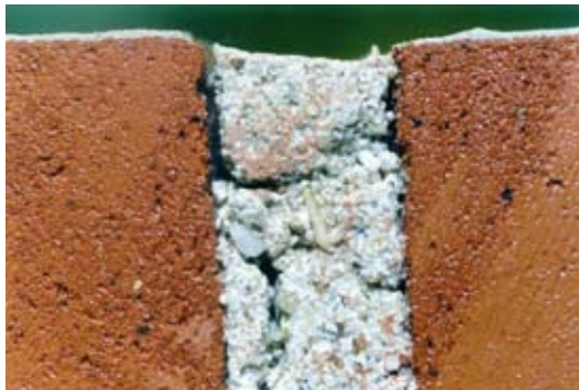
'Traditionele' cementvoeg. Conventional cement pointing.
