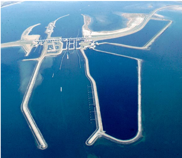
Picture 10.6 Salt-/fresh separation lock in the Philipsdam.
